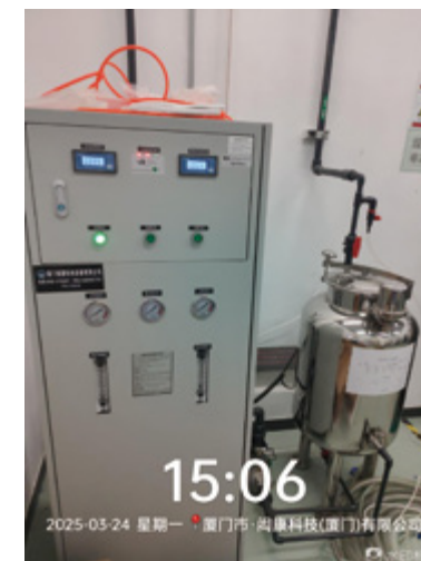
Figure. Renovation of water storage facilities in Xiamen, China.
