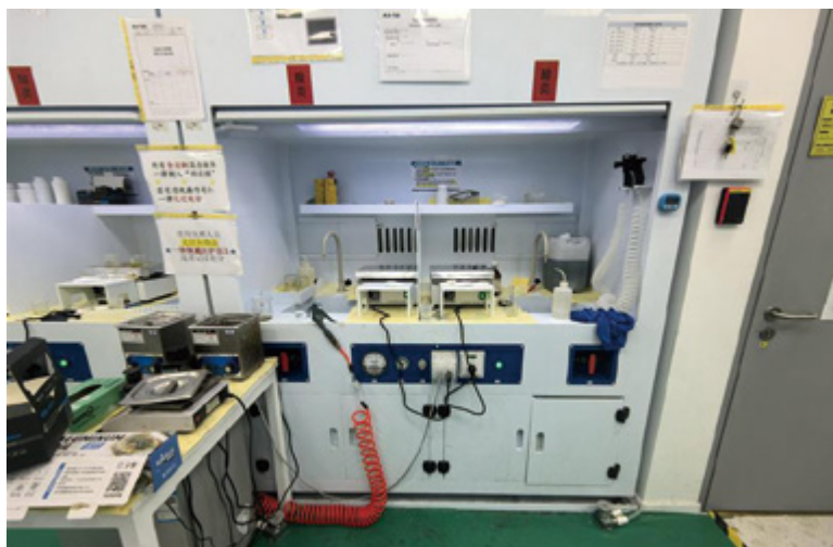
Figure. Shanghai Laboratories foot-operated water control valve
